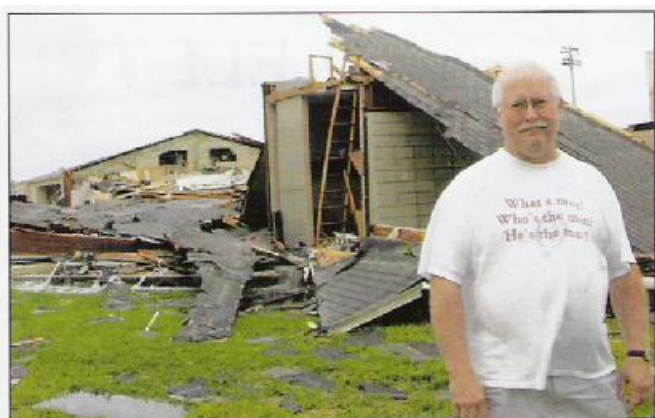
Rev. Stephen K. Wipperman stands in front of the rubble of what had been the church where he is pastor, Our Savior Lutheran Church in Lake Worth, Fla. The building was the only Synod church completely destroyed by Hurricane Wilma.
