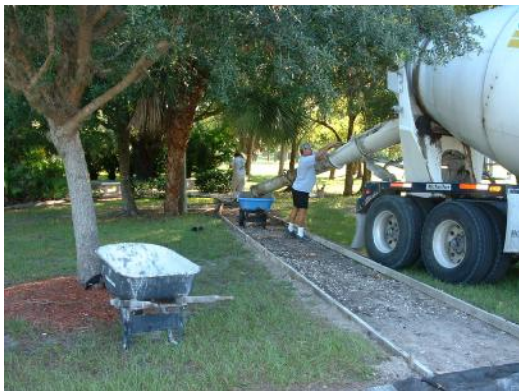
Concrete contractor installing walkway 9/13/07
